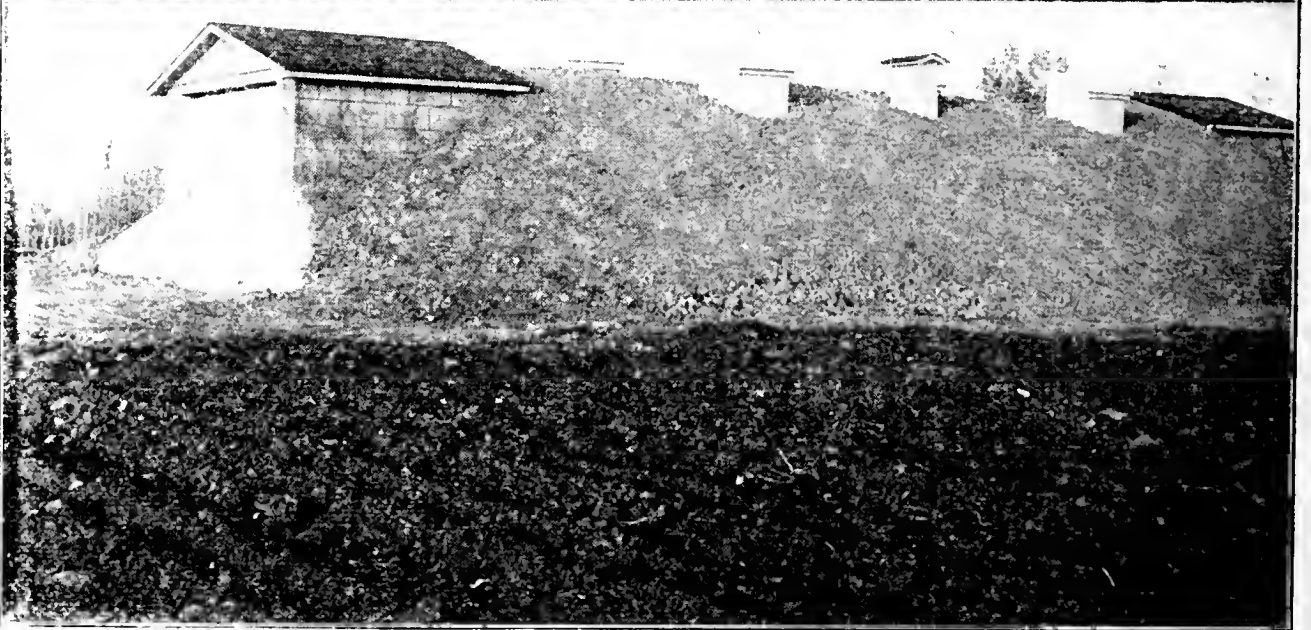
PLATE XVIII.—Getting the Station Cellar Ready for Straw. End and Side Views of Completed Cellar. Photo by Sackett.
